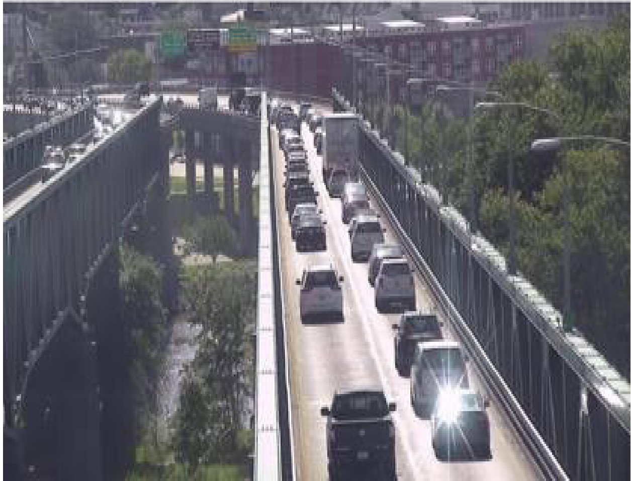
South I-74 @ Toll Plaza to IL (QCTV06) 09/17/2018 12:38:02
